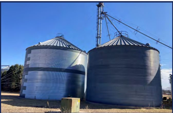
West 48' Storage Bins
