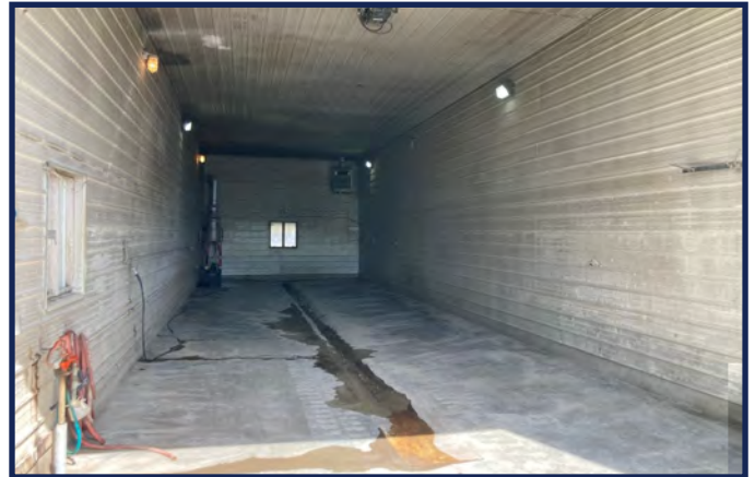
Interior Wash Bay
