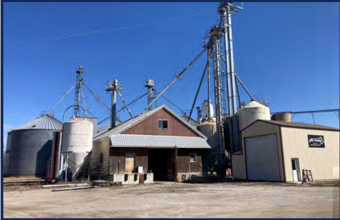
Grain Setup / Feed Facility
