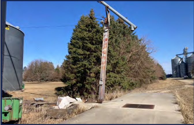
Load-Out / Receiving Pit
