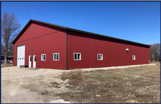
Insulated Shop South / East Sides
