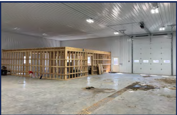
Framed Office Area in Insulated Shop
