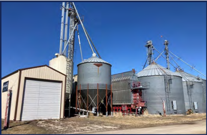
SE Corner of Grain Facility Looking NW
