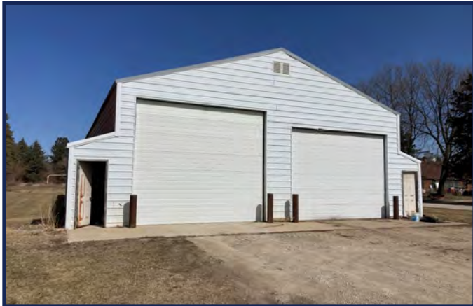
Exterior Wash Building
