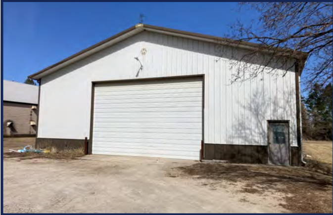
Exterior Storage Shed
