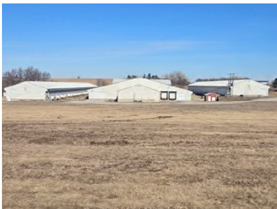
Exterior view looking north
