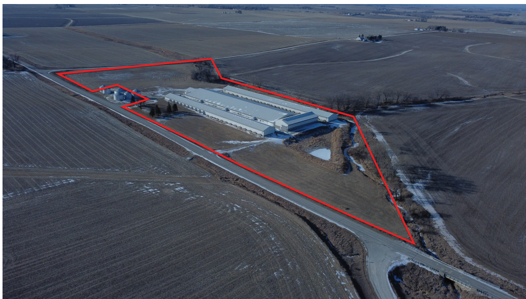
View from the northeast looking southwest
