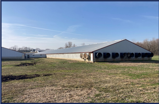
Original Gestation Building
