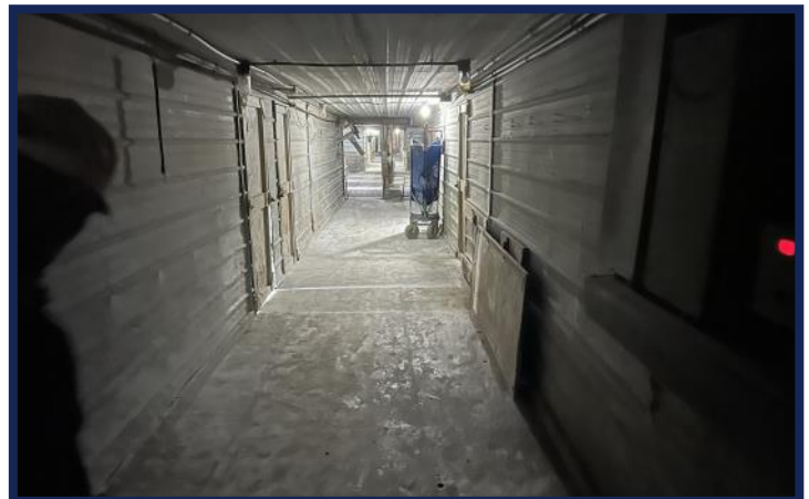
Interior Connecting Hallway
