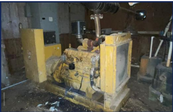
Generator with 8.1L John Deere Engine
