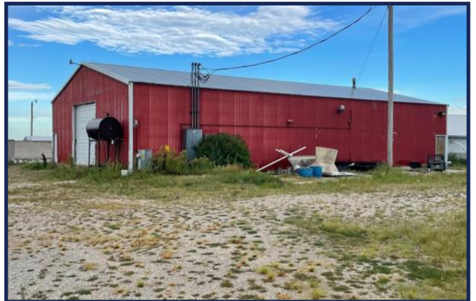
44' X 70' Machine Shed
