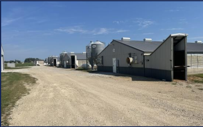
5,400 Head Site SW Looking NE
