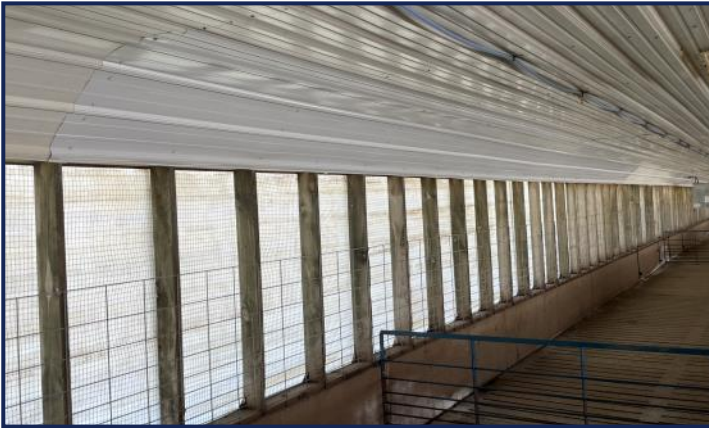
Ceiling Repair Example 2000 Barns
