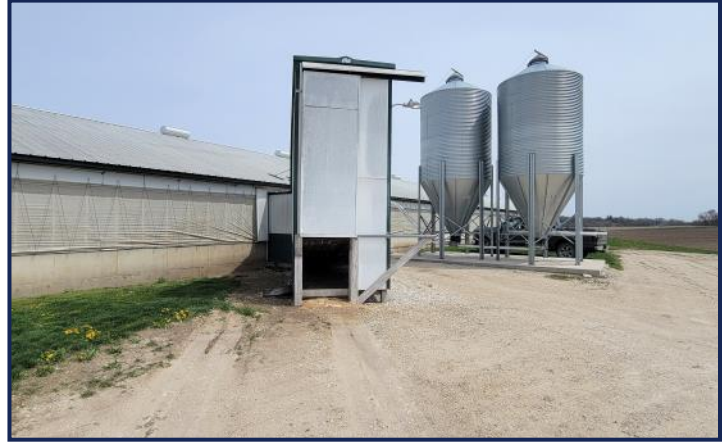
Stationary Load Out and Bins
