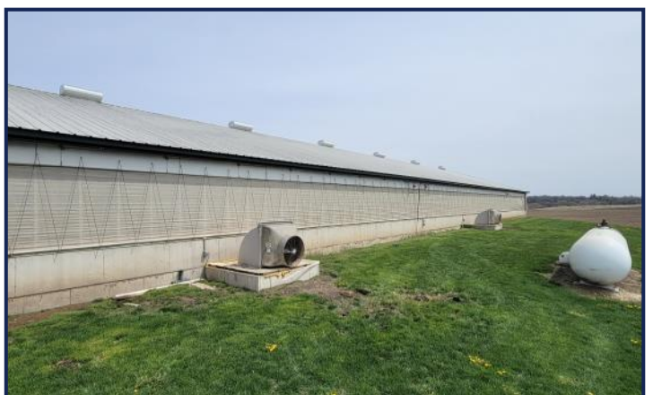
South Curtain and LP Tank (2)
