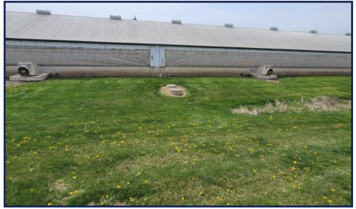
North Curtain and Roof
