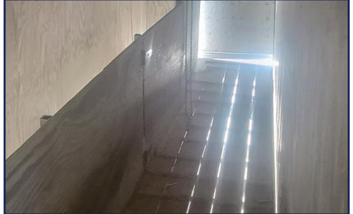
Load Out Interior
