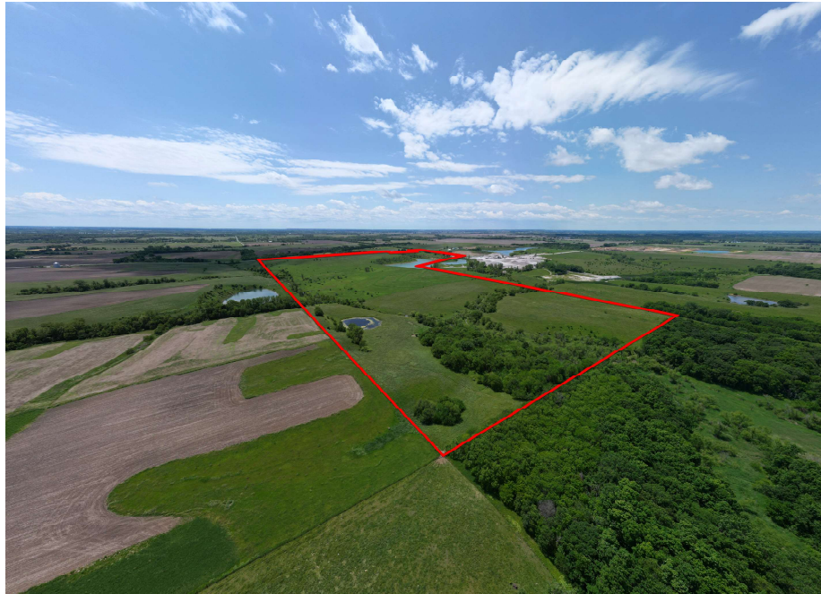
Northeast corner looking southwest
