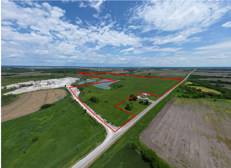
Southwest corner looking northeast
