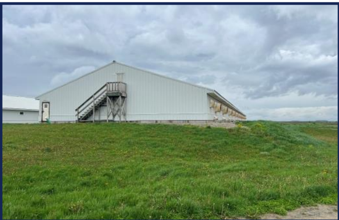
West Farrow Building
