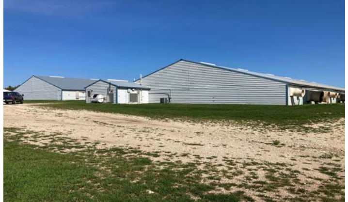
Swine Buildings View from SE
