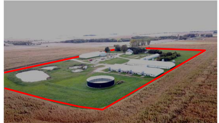
Site View from NE
