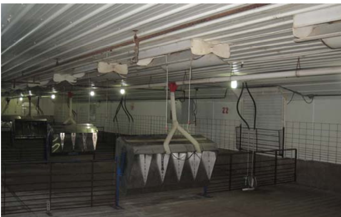
View of Rooms
